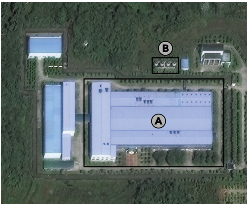
Figure 5: Emeishan CEP3 of plant 814 near Emeishan city. Label A: Enrichment building; B: Cooling towers. Satellite image from 5 October 2014 (Coordinates: 29°38'38.70" N/103°29'25.12" E). © DigitalGlobe. Reproduced by permission of DigitalGlobe. Permission to reuse must be obtained from the rightsholder.
