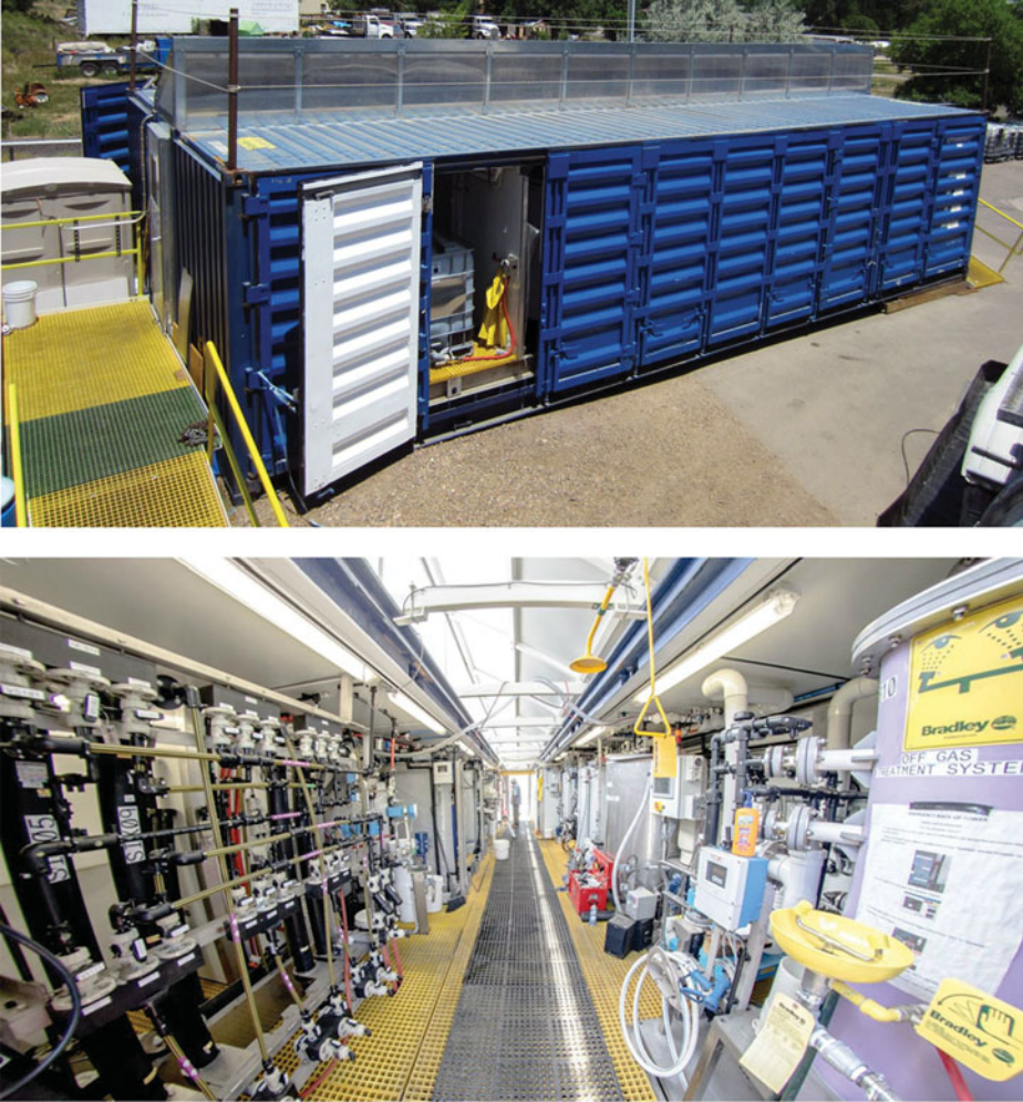
Figure 3. Urtek LLC uranium extraction pilot plant (Urtek LLC).
