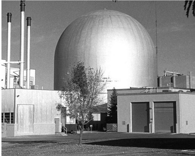
Figure 2: Experimental Breeder Reactor-II. Source: Argonne National Laboratory.
