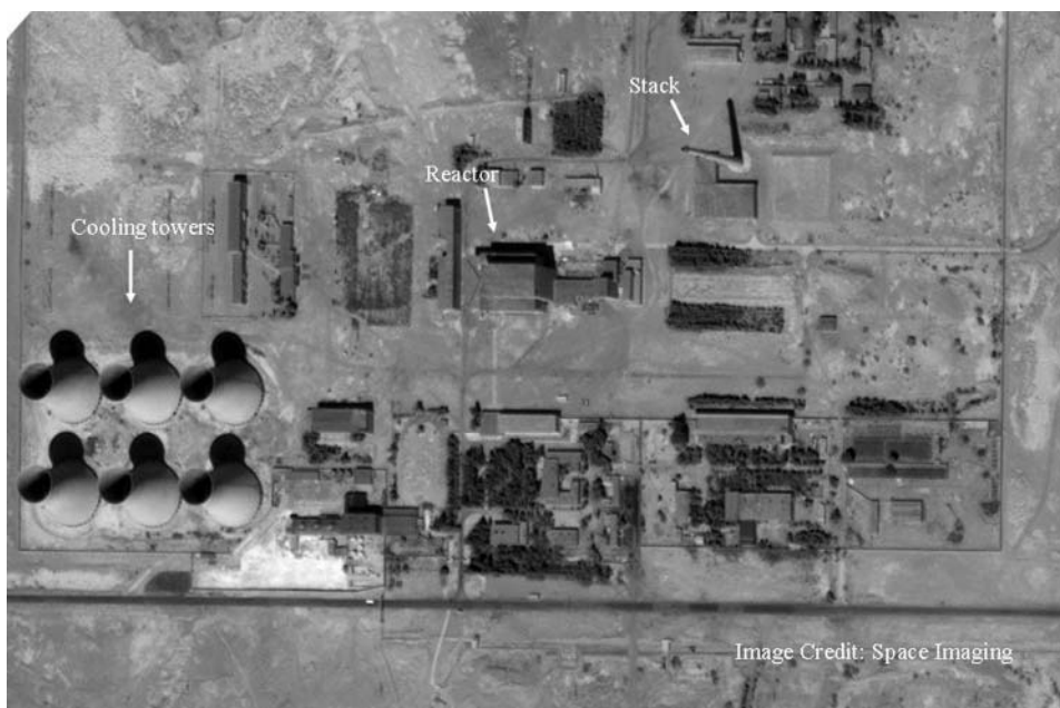
Figure 4: The Jiuquan plutonium production reactor. The image is from 25 February 2004. (Coordinate: 40° 13'23.32"N/97°21'21.26" E). Source: Space Imaging.
